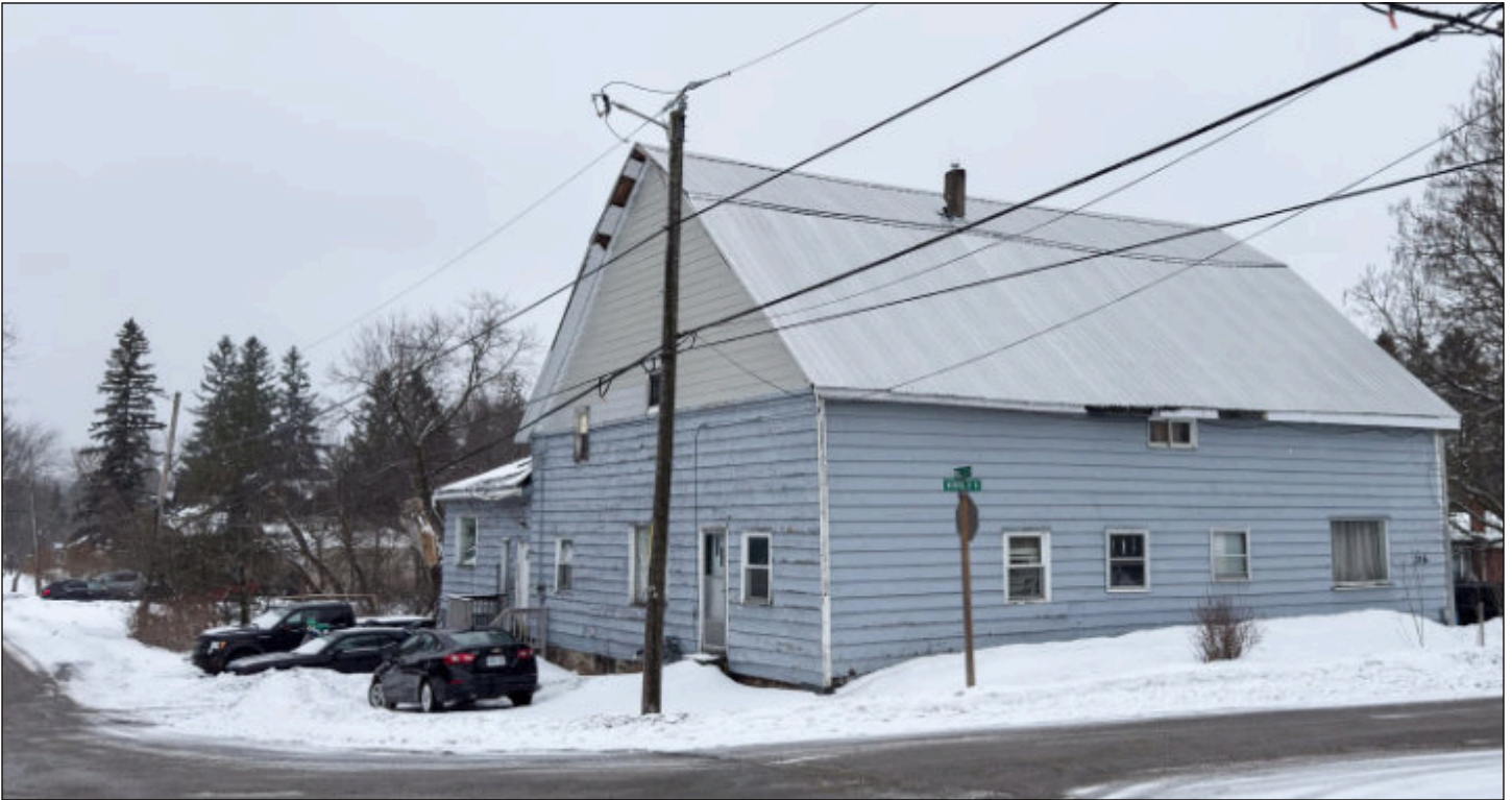
The original barn on Mill Street North where the Bierstiekers and Wagenaars lived and Newcastle Cement Block began in the basement. Photo: Paddy Duncan
