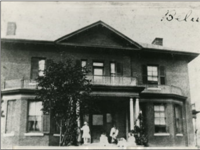
Belmont House early 1900s - note double posts on porch and wooden railing on upper balconies. Porch posts were altered by 1940, and upper railings removed.
