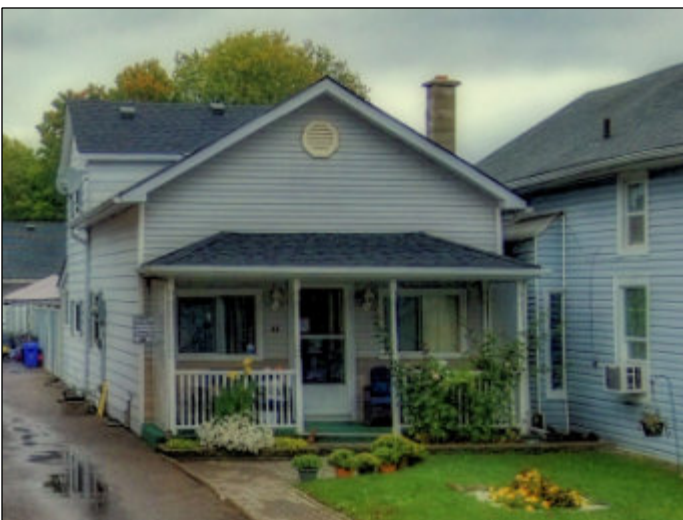
Joseph Atkinson's home at 44 King Ave. E., in Newcastle from 1866-1884. It now has new(er) siding and a front porch, but the structure is largely unchanged.
